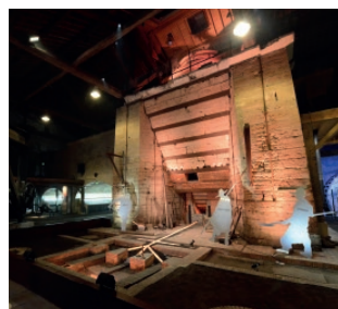
Haut-Fourneau - Metallurgic Park
